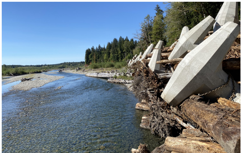
Completed Engineered Log Jams at MP 3.5
