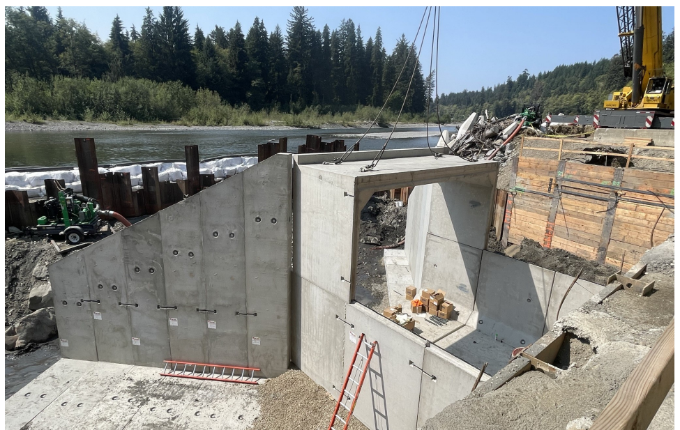
Placement of the MP 4 Box Culvert outlet sections
