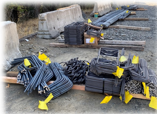
East tunnel portal structure material
