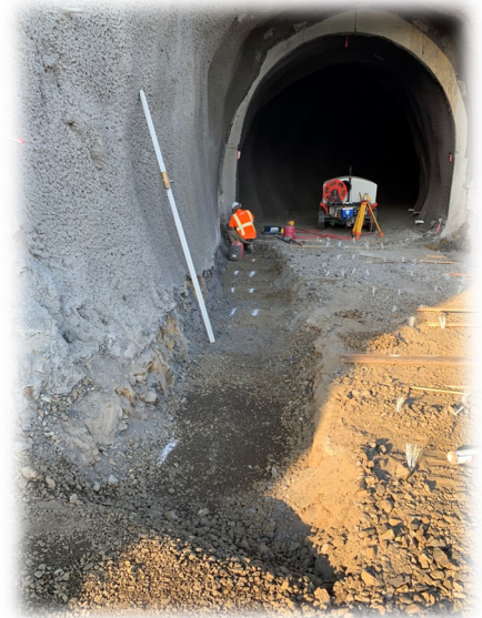
East tunnel portal footing layout
