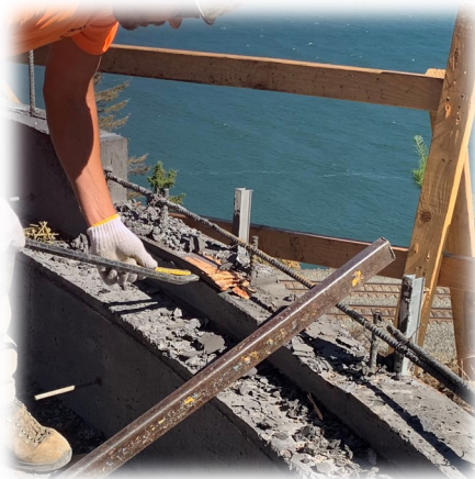
Below: Striping concrete form-work at East Bench outlook
