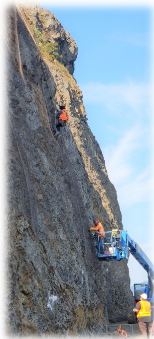
Left: Rockfall fence installation
