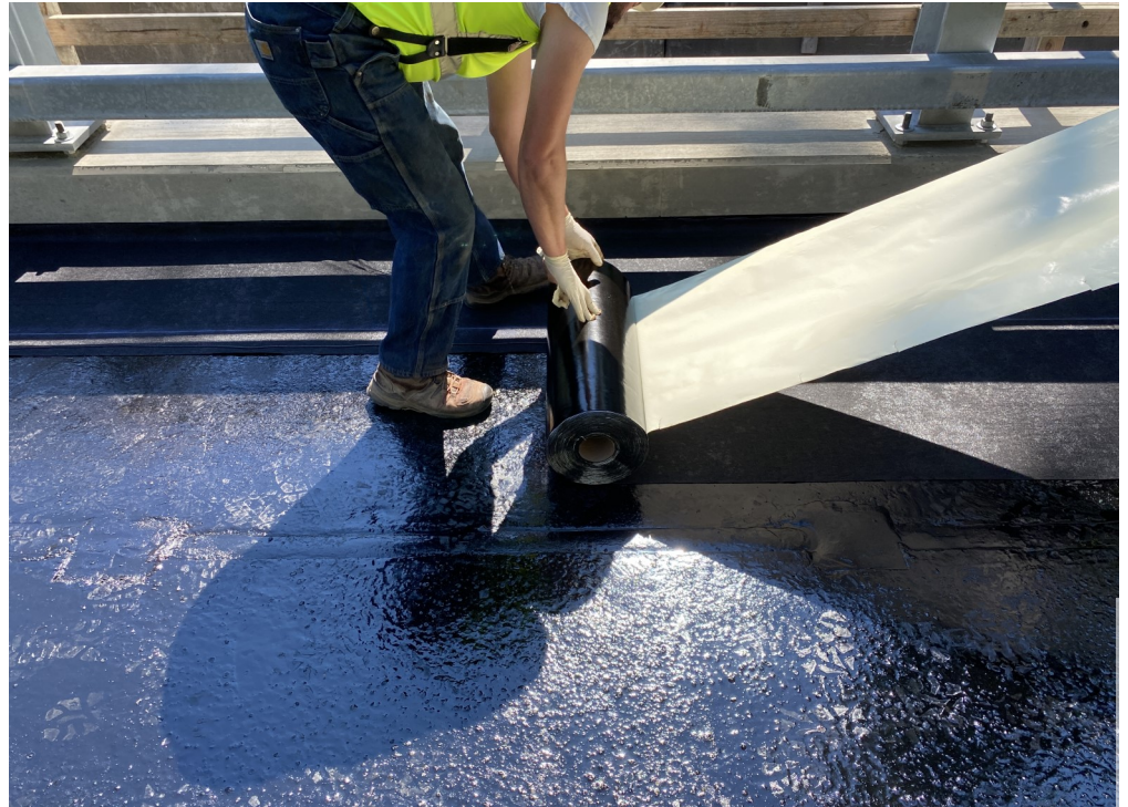
Placing the waterproofing membrane on the primed bridge deck surface
