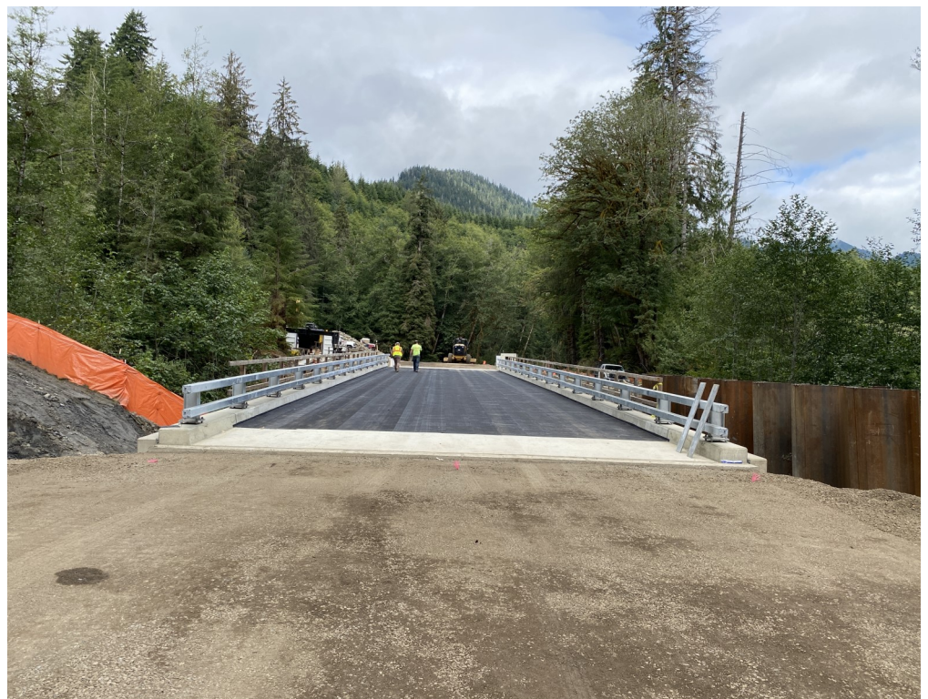
Roadway aggregate graded to the bridge prior to asphalt paving on 8/29
