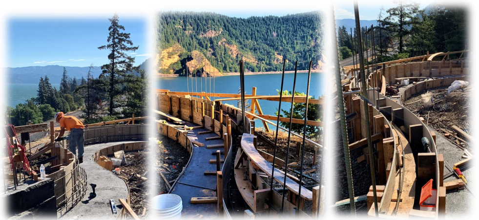
Three below: East Bench structure concrete form and rebar
