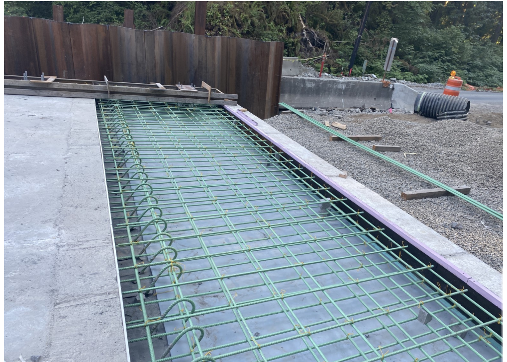
Rebar for the west Tower Creek approach slab
