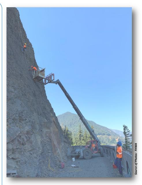
Rockfall Protection; Contour Pin Installation at Mid Slope
