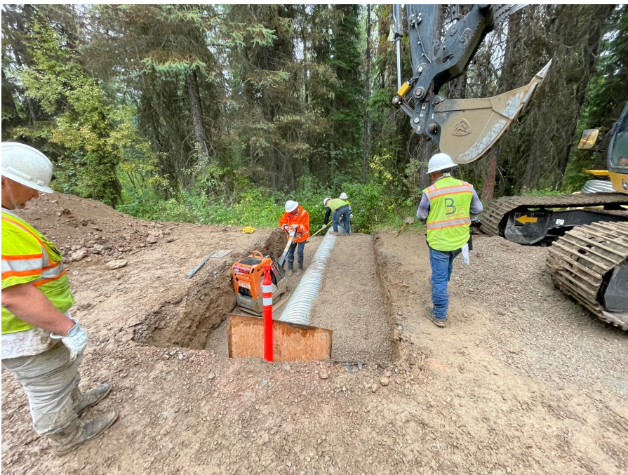
Installing 24" Culvert at N. Fork Road
