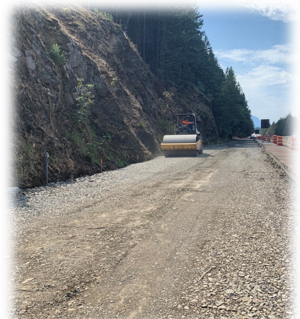
Compacting subgrade
