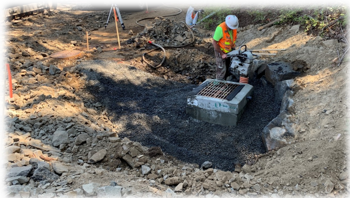
Below: Backfilling around an inlet
