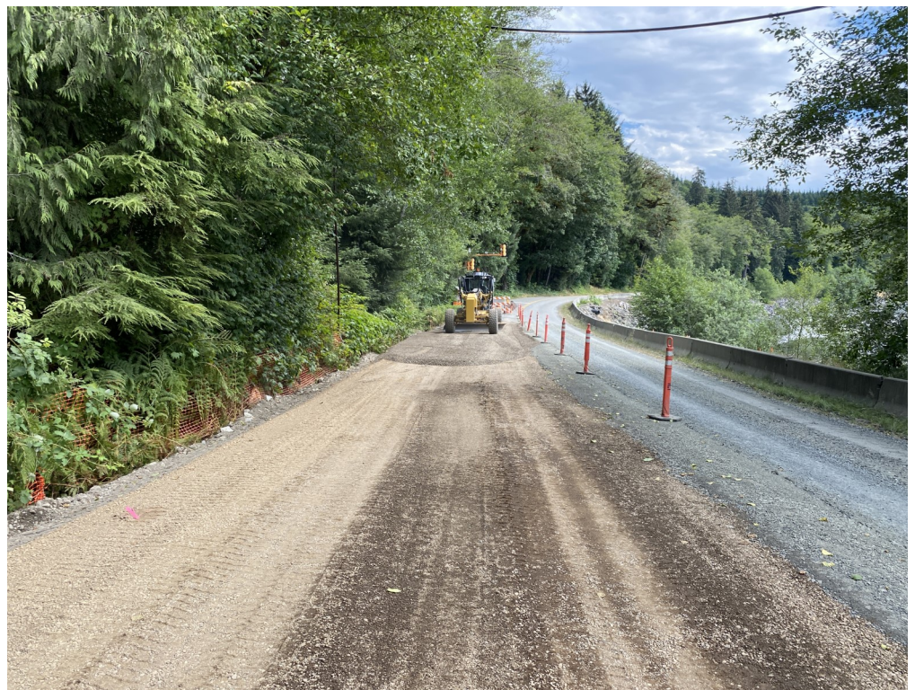
Grading the roadway approaches to the Tower Creek bridge
