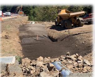
Water Quality Swale Drain Rock Wrapped in Geotextile Filter
