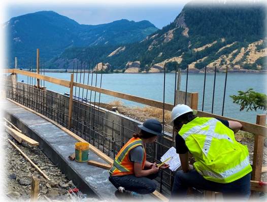
Concrete wall rebar inspection
