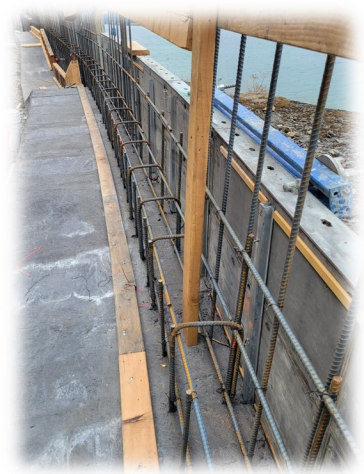
Retaining wall reinforcement on East Bench
