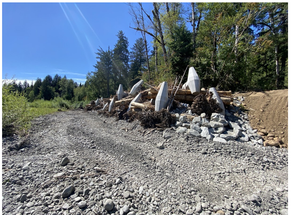
Completed ELJ unit at MP 3.5
