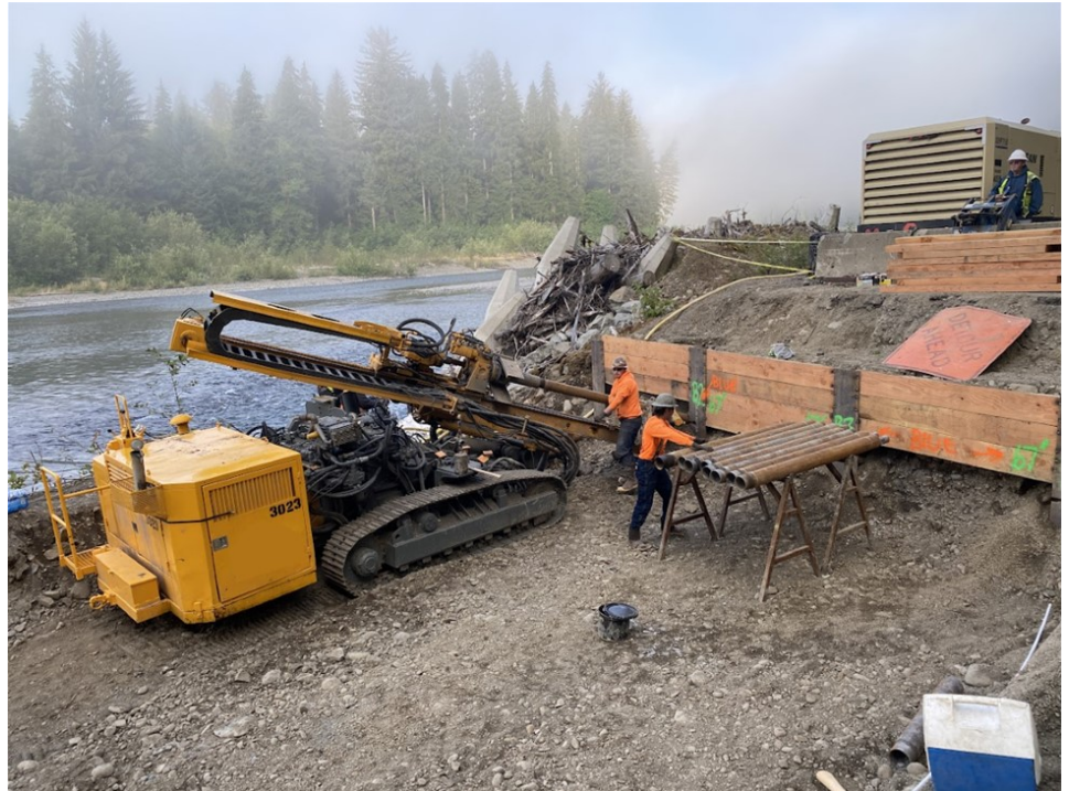
Condon Johnson drilling tieback anchors at MP 4
