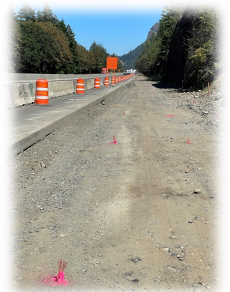
Below: Staking subgrade
