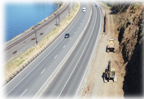
Excavation for water quality drainage swale
