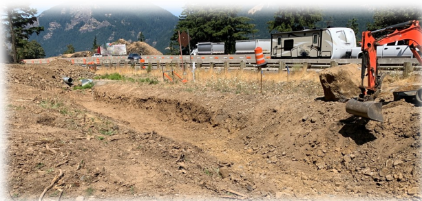
Excavation for water quality drainage swale
