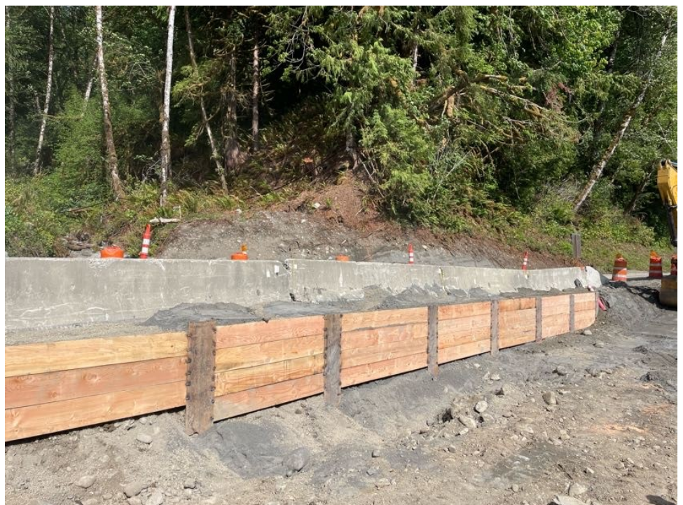
Start of timber lagging for temporary shoring at MP 4
