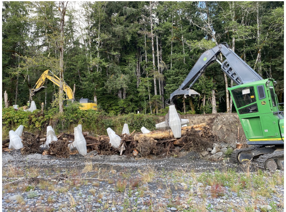
Installation of ELJ units at MP 3.5
