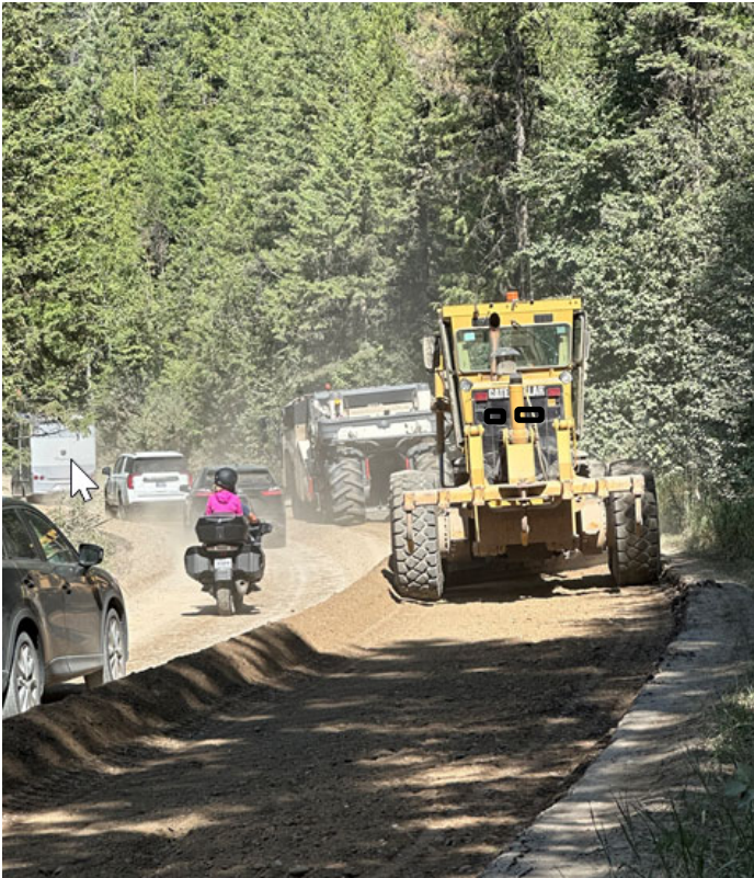
Pulverizing (FDR) and Blading the GTSR
