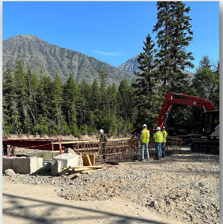
Abutment 1—Tying Rebar for Pile Cap
