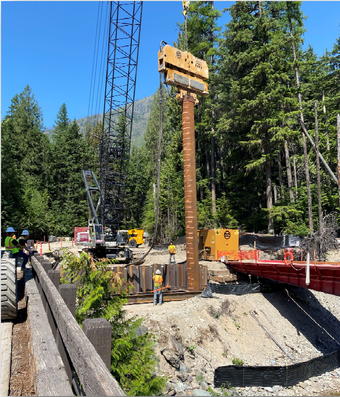
Driving test pile at Abutment 2
