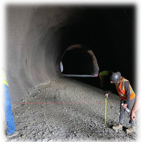
Checking tunnel subgrade at Adit #4
