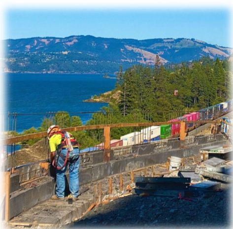
Concrete cured and forms removed
