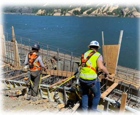
Forming wall footing
