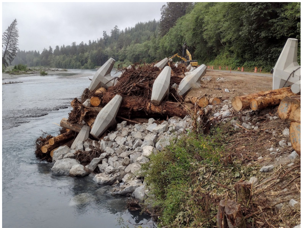
The upstream end of the complete ELJ #18
