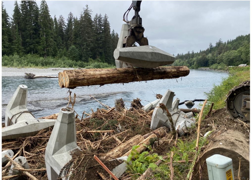
ICI constructing Engineered Log Jam #16 at MP 4
