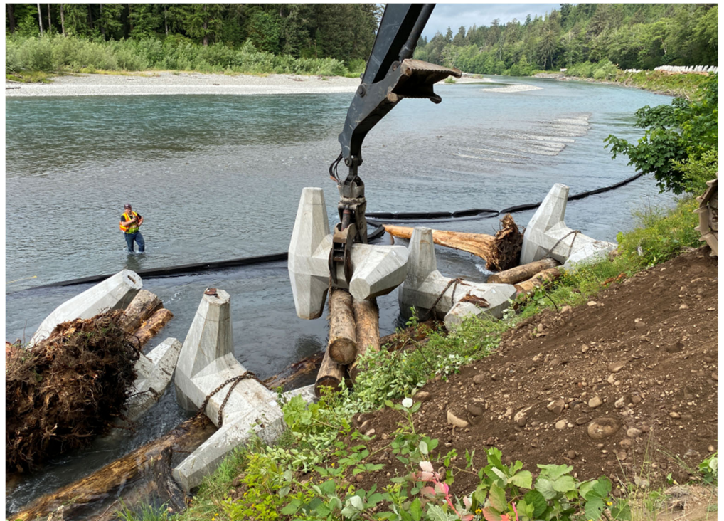
ICI constructing an Engineered Log Jam at MP 4
