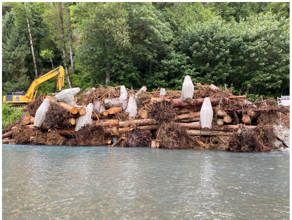
The first completed Engineered Log Jam of 2022
