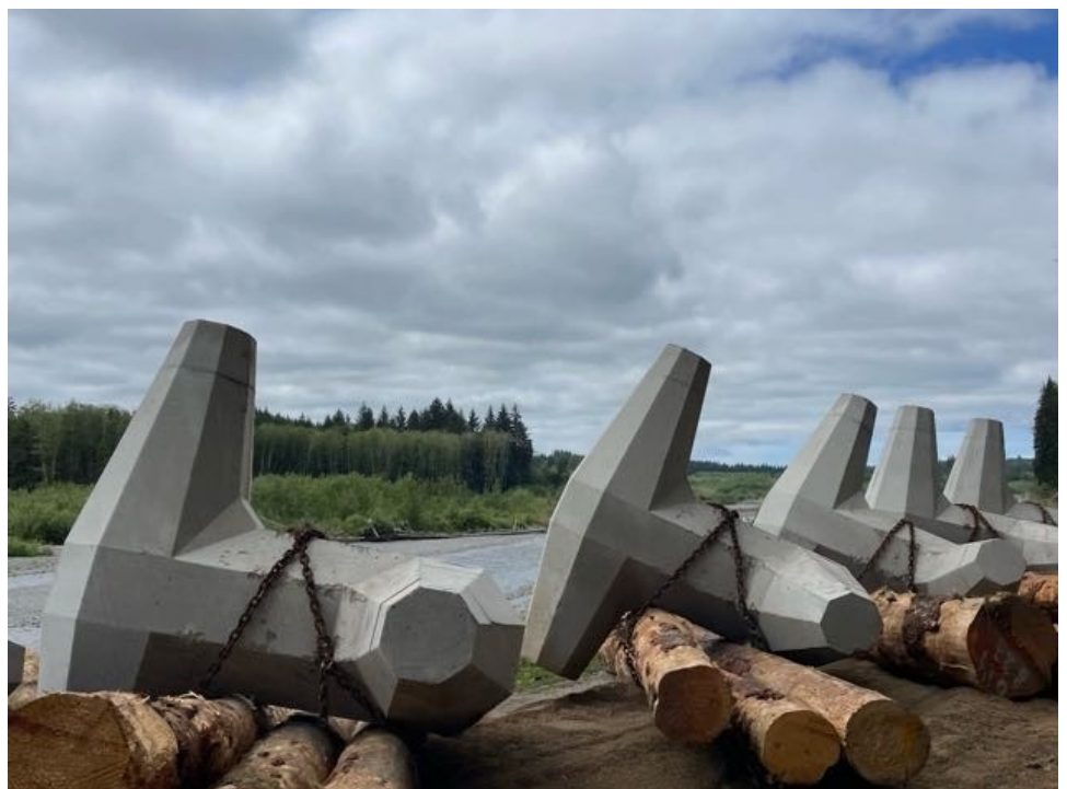
Pre-assembled Engineered Log Jams at MP 3.5
