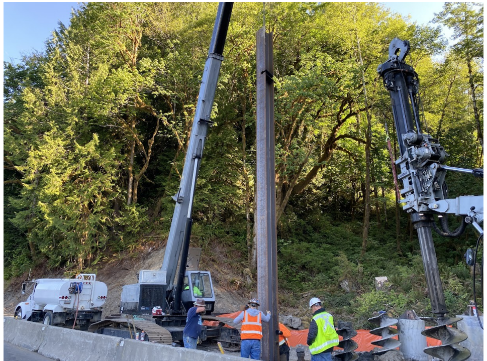
Installing soldier piles performed by Versatile Drilling at MP 4.0
