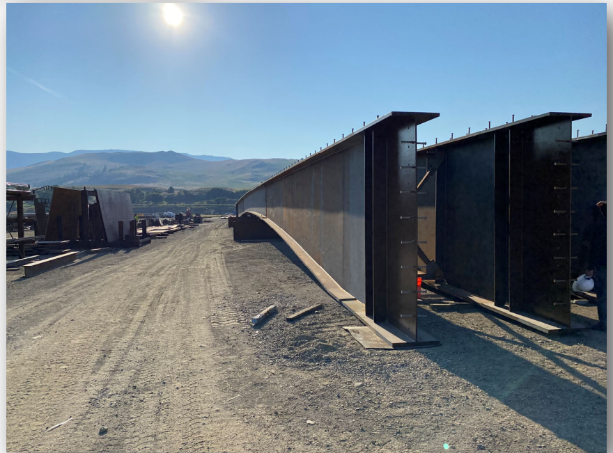
Completed Girders at Fabrication
