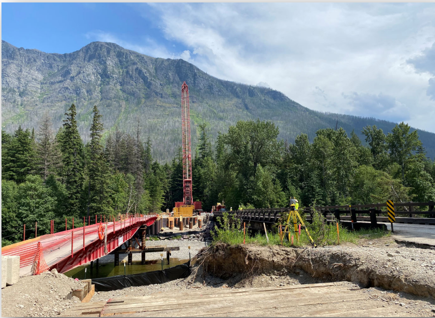
Piles at Abutment 1 Complete
