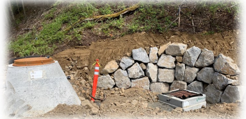
Rockery wall at drop inlet
