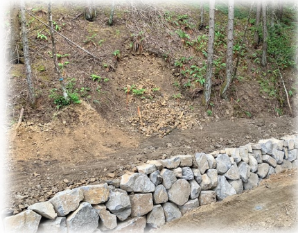
Installation of mid-slope attenuator bases
