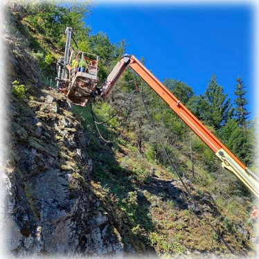
Installation of mid-slope attenuator bases
