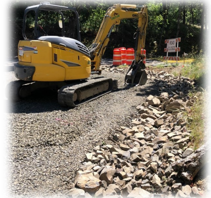
Below: Riprap installed
