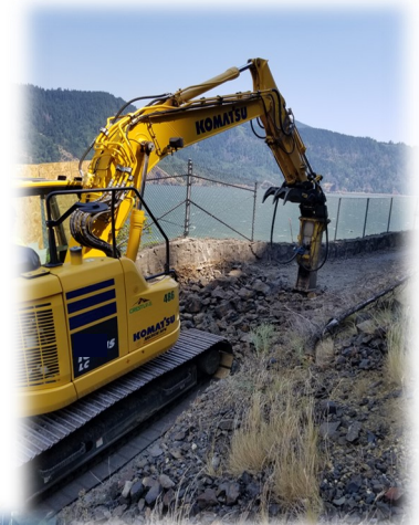
Left & Below: Dry swale—filling the holes with rock
