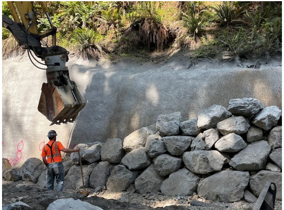
Construction of the Rockery Facing
