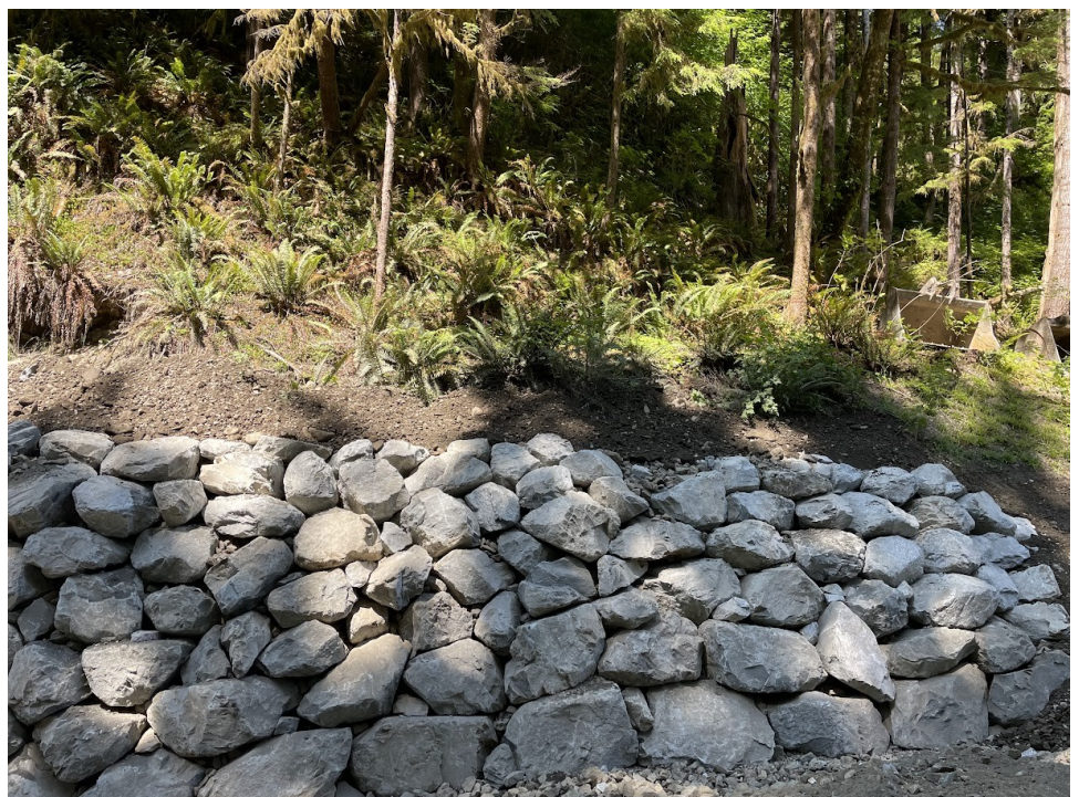
Completed East end of the Soil Nail Retaining Wall and Rockery
