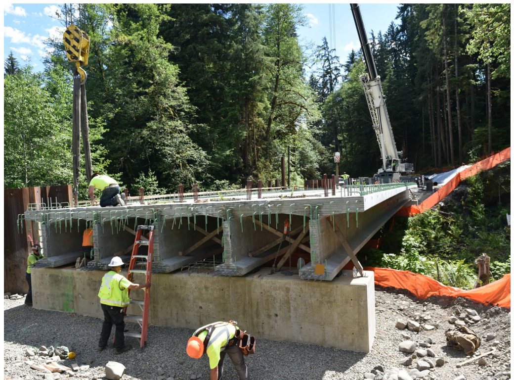
ICI installing new prestressed bridge girders at Tower Creek
