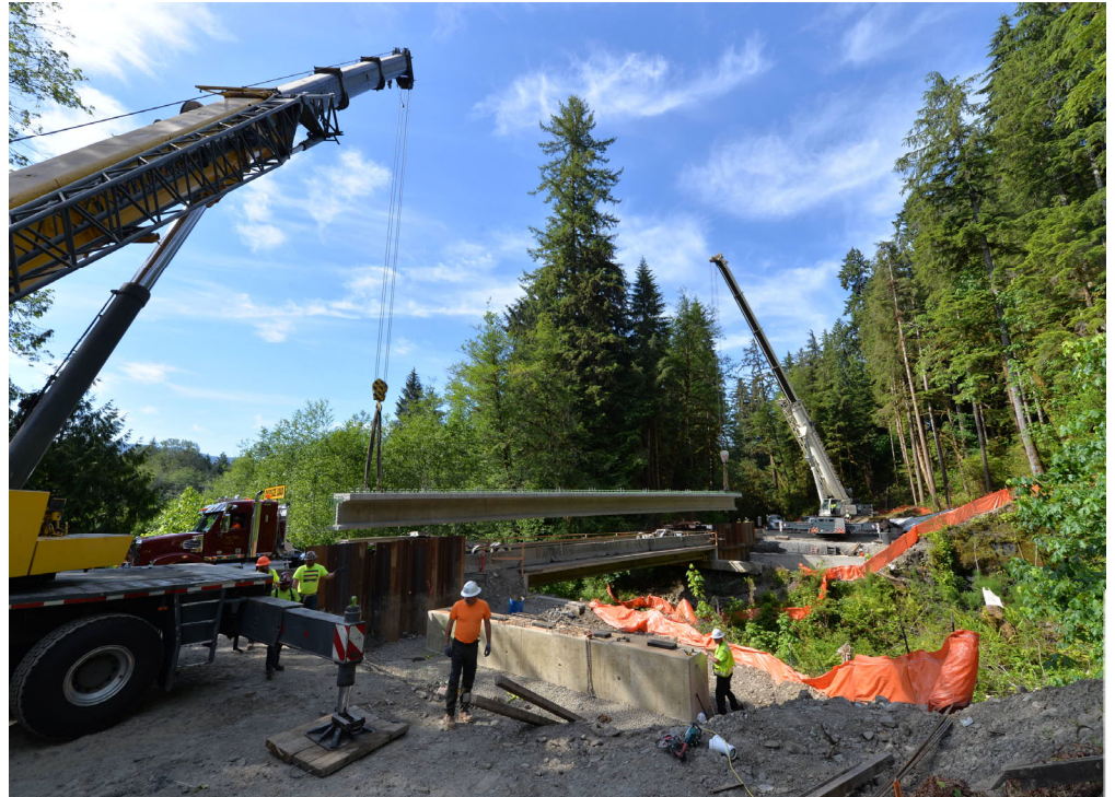
ICI installing new prestressed bridge girders at Tower Creek
