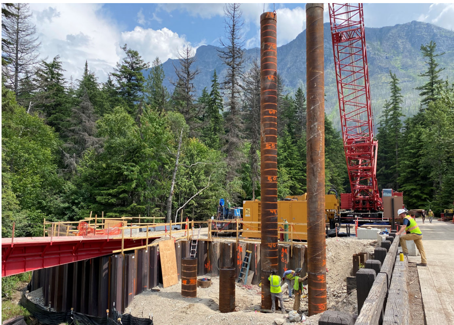
Splicing piles at Abutment 1
