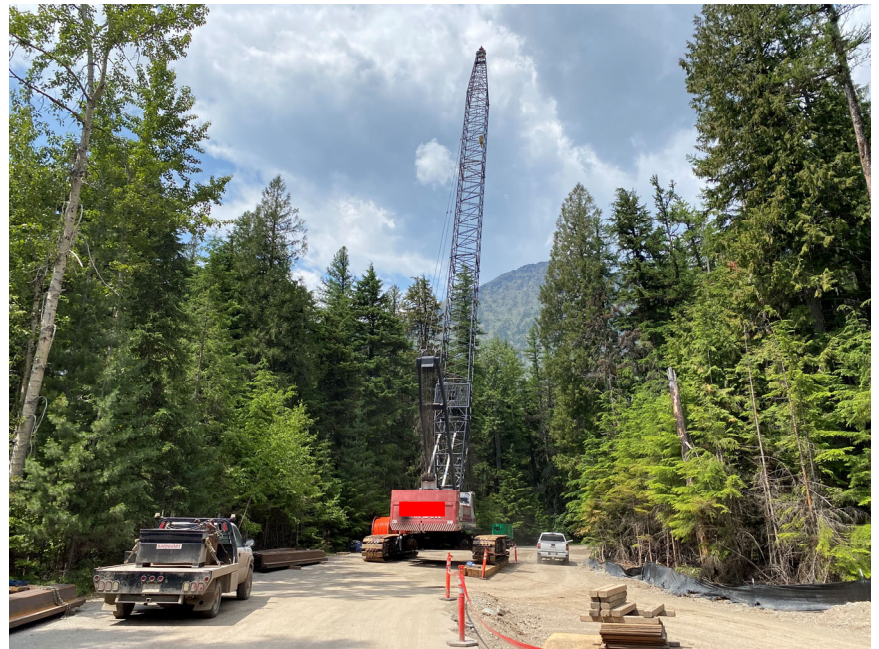
250 ton crane erected on west side of bridge
