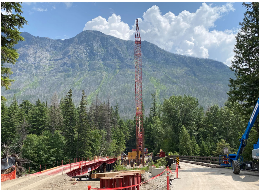
Temporary Bridge Installed
