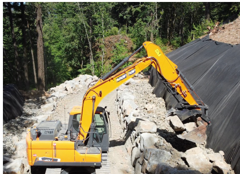
Preparation for rockery placement at Nature Wall
