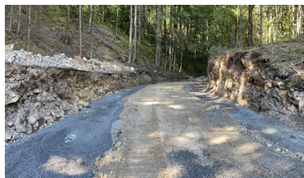
Preparation for rockery placement at Nature Wall
