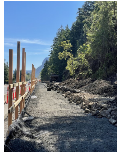
Staging rocks for rockery wall at Nature Wall
