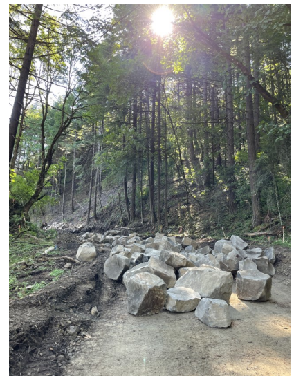
Staging rocks for rockery wall at Nature Wall
