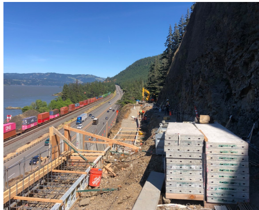
East Wall W2 Excavation and Formwork
