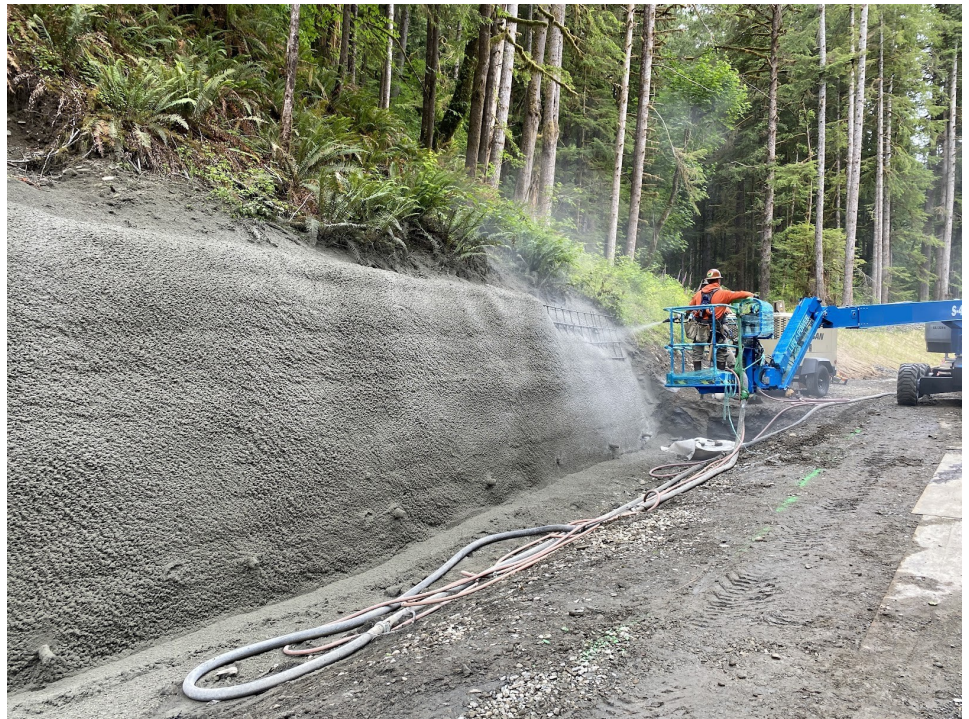
Exterior layer of Shotcrete being applied
