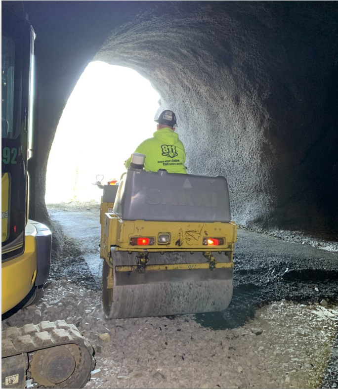
Tunnel Grading and Compaction in Adit
