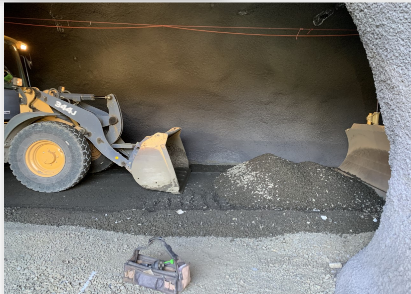
Tunnel Grading and Aggregate
