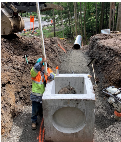
Setting stormwater drainage inlet basin
