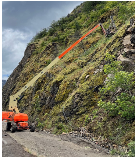
Drilling mid-slope attenuator anchors
