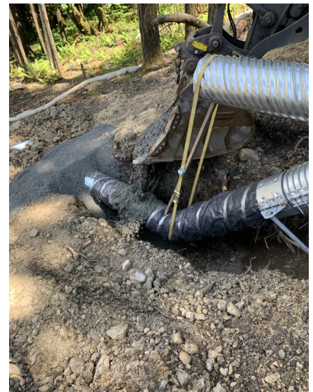
Placing concrete for drop culvert thrust block
