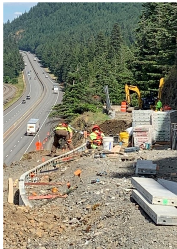
Ongoing Excavation of East Side Retaining Wall
