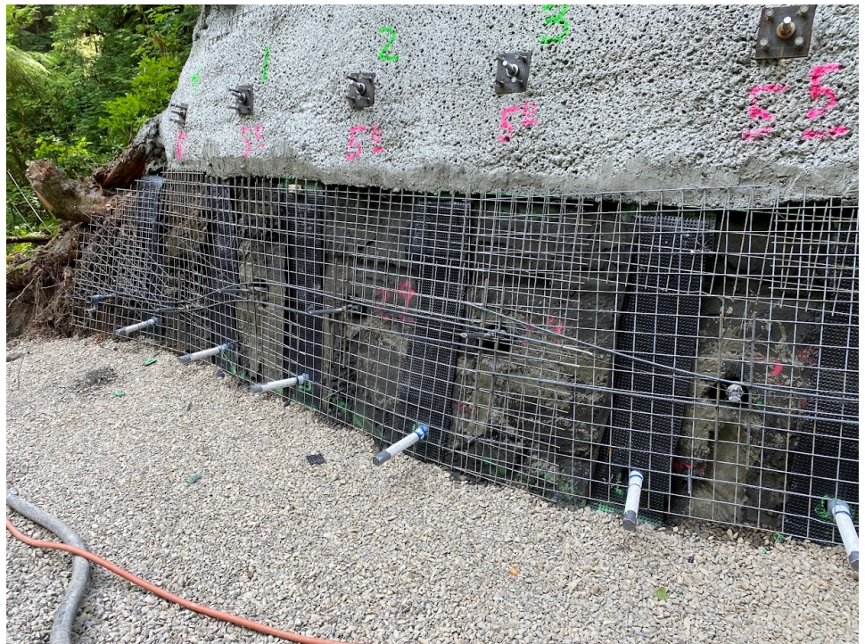
Reinforcing steel, drainage sheets, and weep holes beneath Shotcrete
