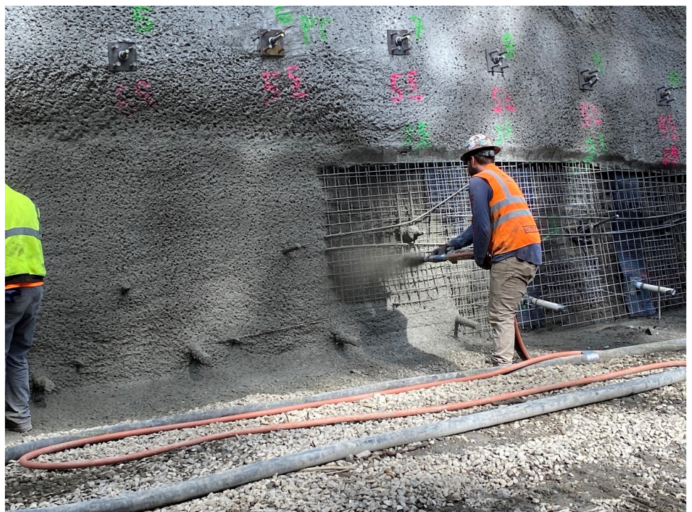
Application of the interior layer of Shotcrete
