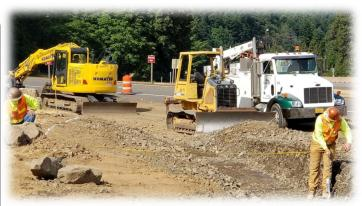
Bio-swale construction, ditch excavation, and material stockpiling. Providing clean runoff waters into the Columbia River.
