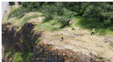
Placement of wire mesh anchors on Stepped Cut
