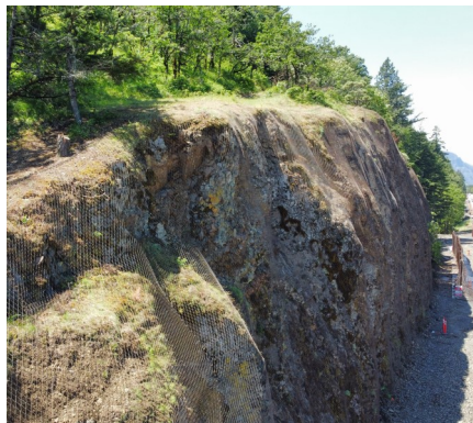
Finished wire mesh at The Pinnacle
