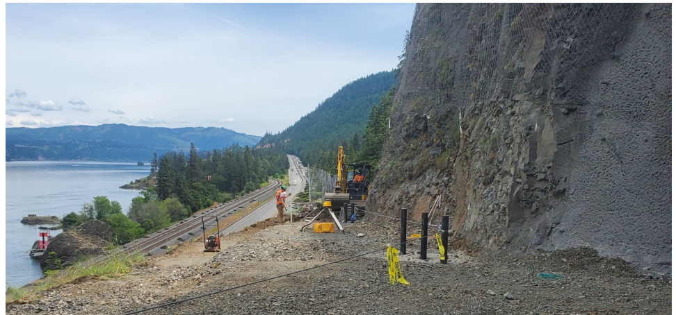
Ongoing Excavation of East Side Retaining Wall
