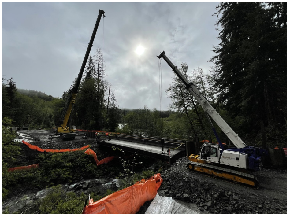
Removal of concrete girder from Tower Creek bridge (Source: FHWA)
