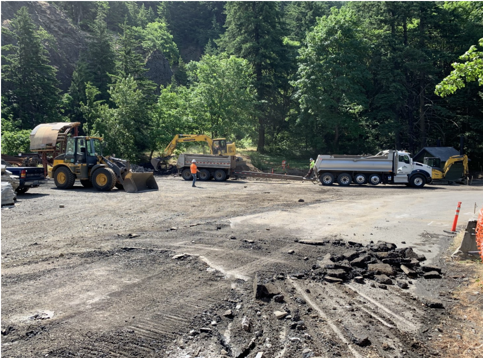
West Parking Lot Asphalt Removal
