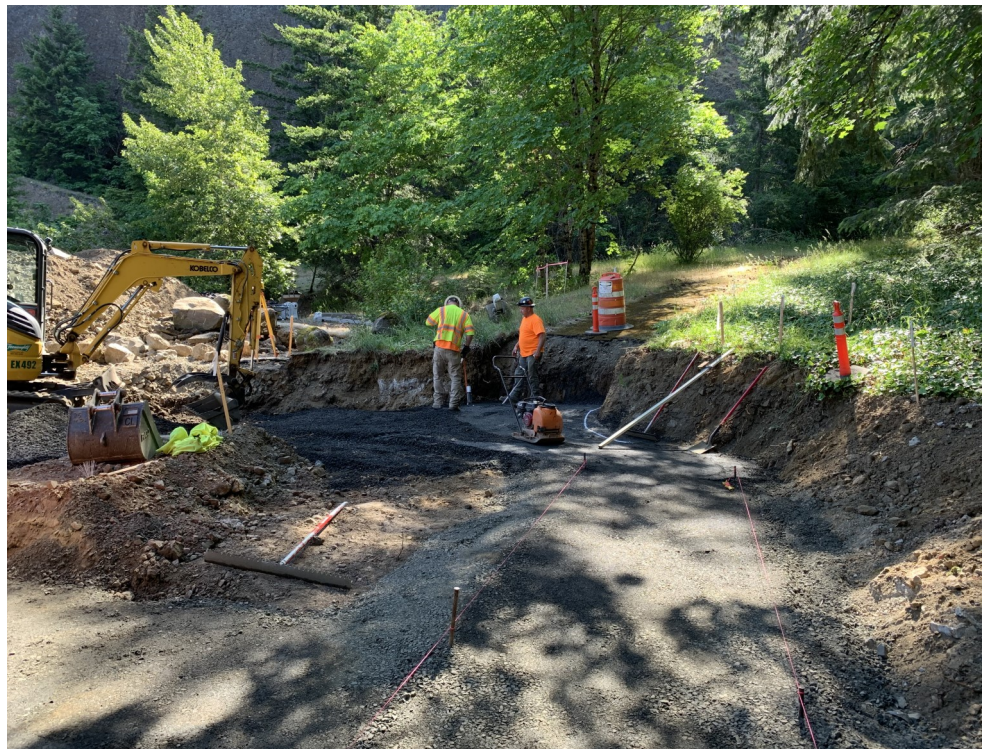
West Trailhead Plaza Sidewalk Construction
