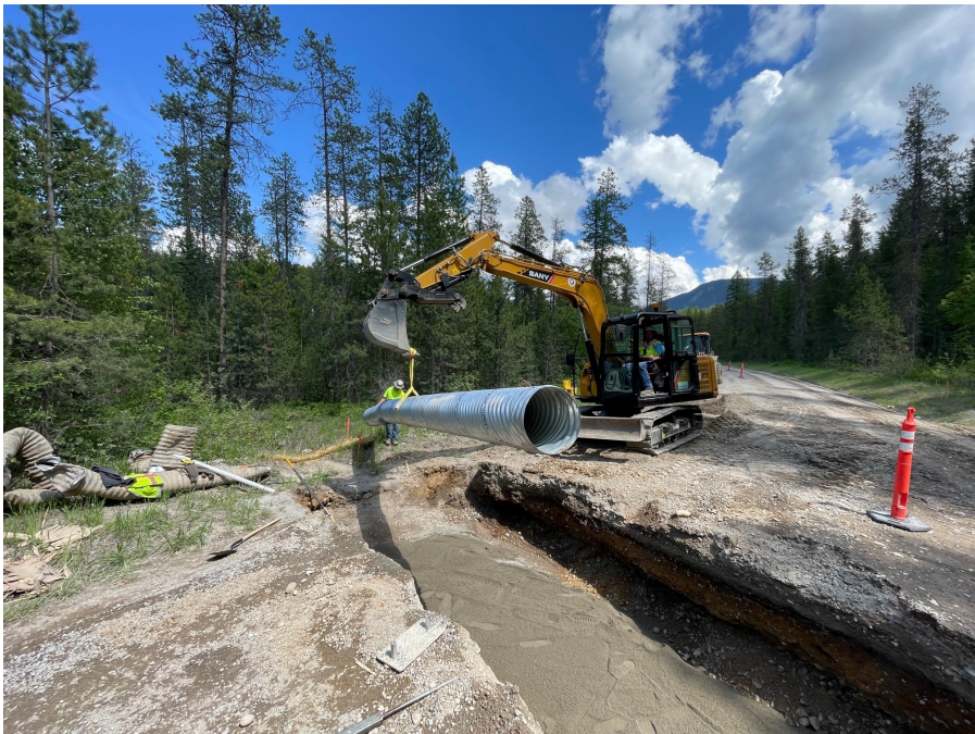
Culvert Installation —Blankenship Road
