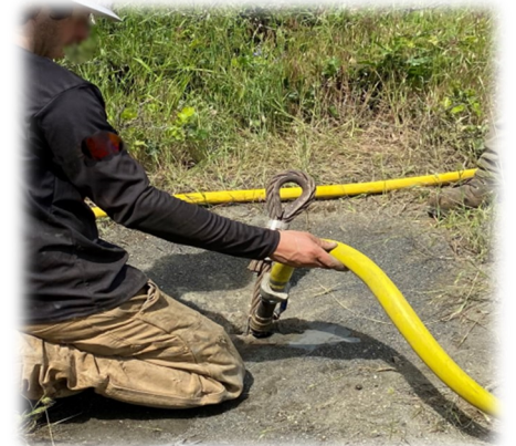
Drilling ground anchors for wire mesh
