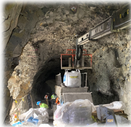
Adit #2 Shotcrete batch plant set up
