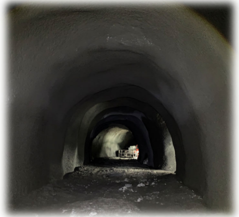
Colored shotcrete between Adit #3 & #4
