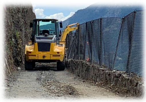
Masonry wall removal at East Bench
