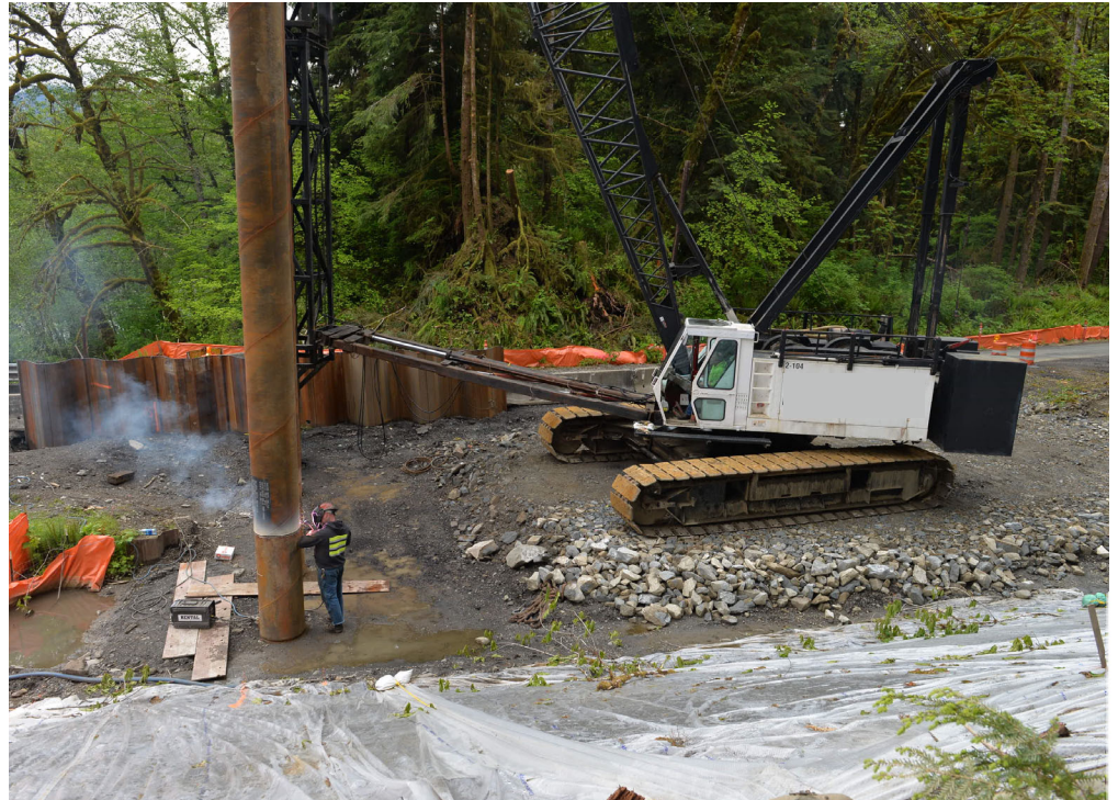
ICl subcontractor Installing 24" steel pile foundation
