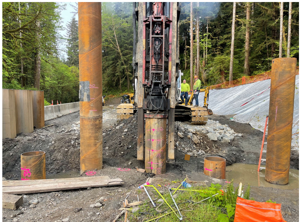
ICl subcontractor Installing 24" steel pile foundation
