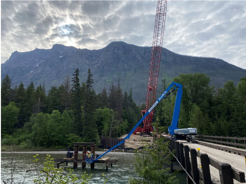
Prepping piles for installation of the Jumper System.
