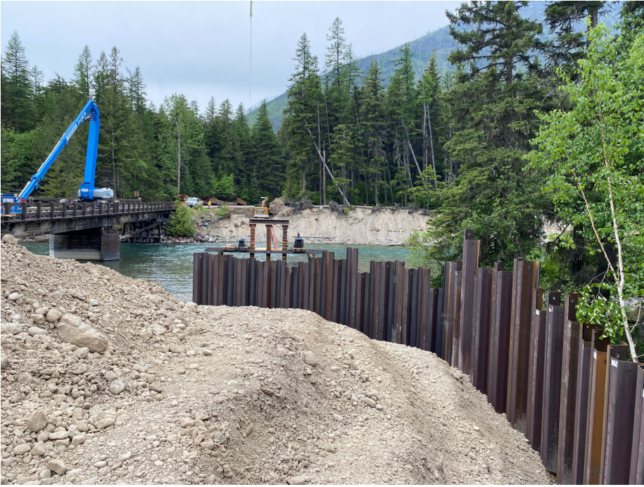
Sheet Pile installed on east end.
