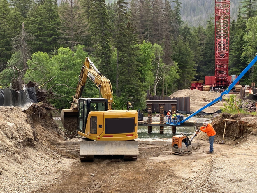
Constructing landing on west end for the Jumper System.
