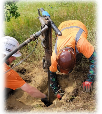
Drilling ground anchors
