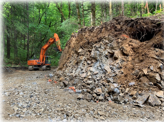
Excavating for the trails and rockery walls
