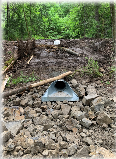
Culvert and rip rap installation
