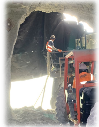
Adit #3 shotcrete curing curtain installation
