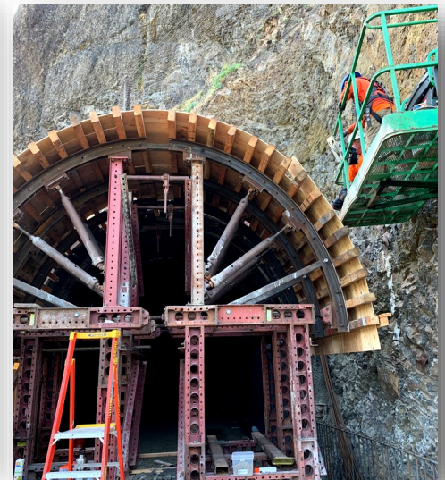
Below: West Portal Concrete Structure Support Assembling
