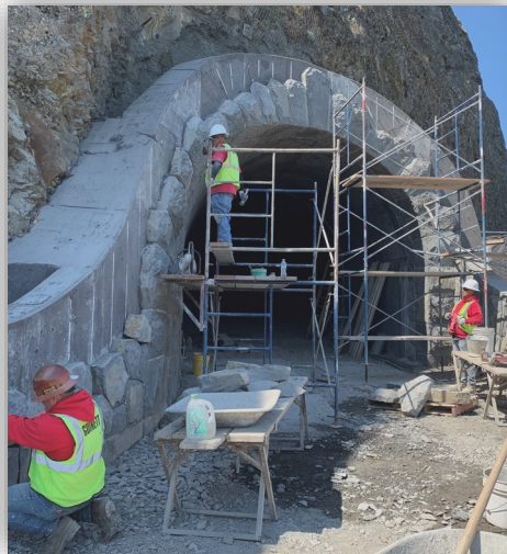
Below: West Portal Concrete Structure Support Assembling
