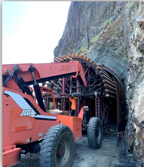
Below: West Portal Concrete Structure Support Assembling
