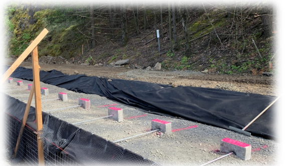
Anchor blocks in MSE wall
