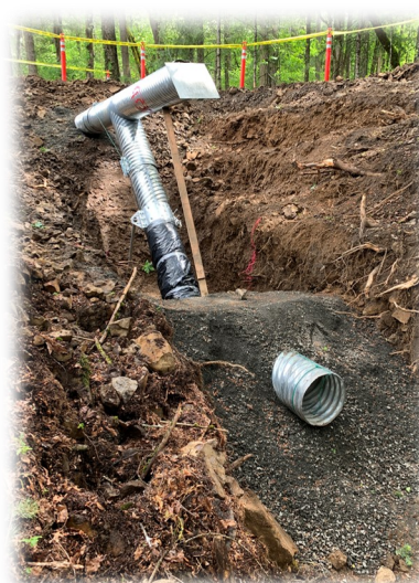
Drop culvert installation
