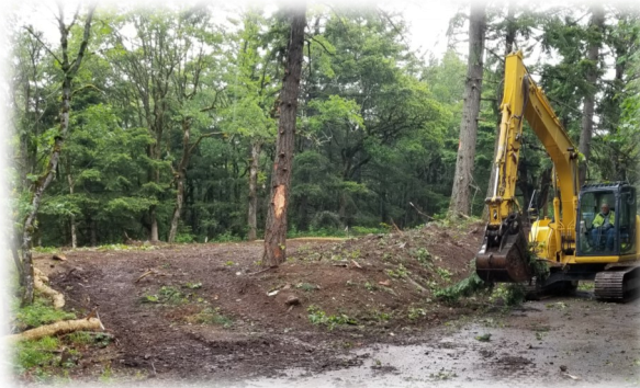
Clearing and grubbing operations continue
